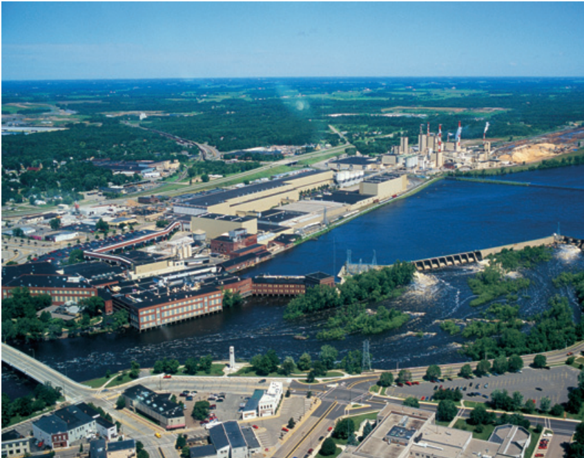
Wisconsin Rapids mill site.
